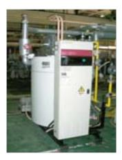
Solvent neutralizer feeder (to prevent oxidation of solvent and handle corrosion of equipment)
